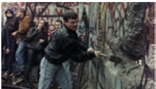
Demolition of Berlin wall
